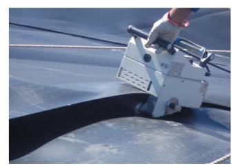
A **HÜRNER** wedge welder HWW 1000 joints a 2.5 mm PE-HD surface lining.
